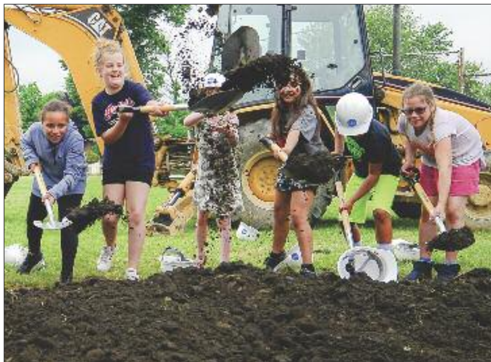
Ely Students throw dirt during the groundbreaking ceremony for their new school.
